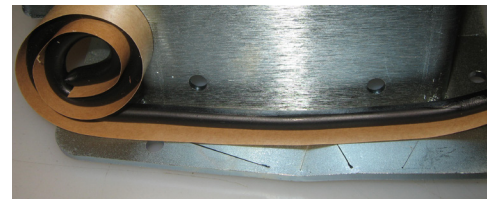
Figure 15: Apply Butyl Tape
