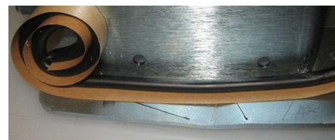
Figure 15: Apply Butyl Tape
