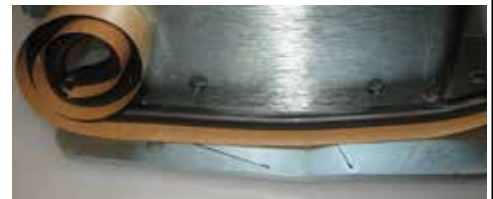
Figure 15: Apply Butyl Tape
