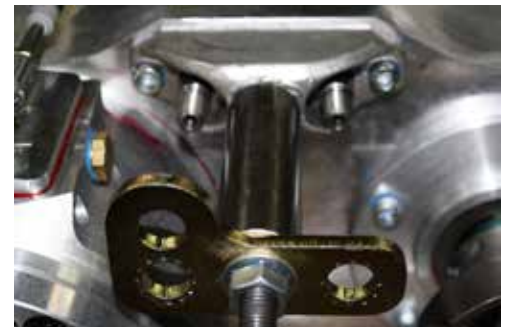
support tube and bracket installed
